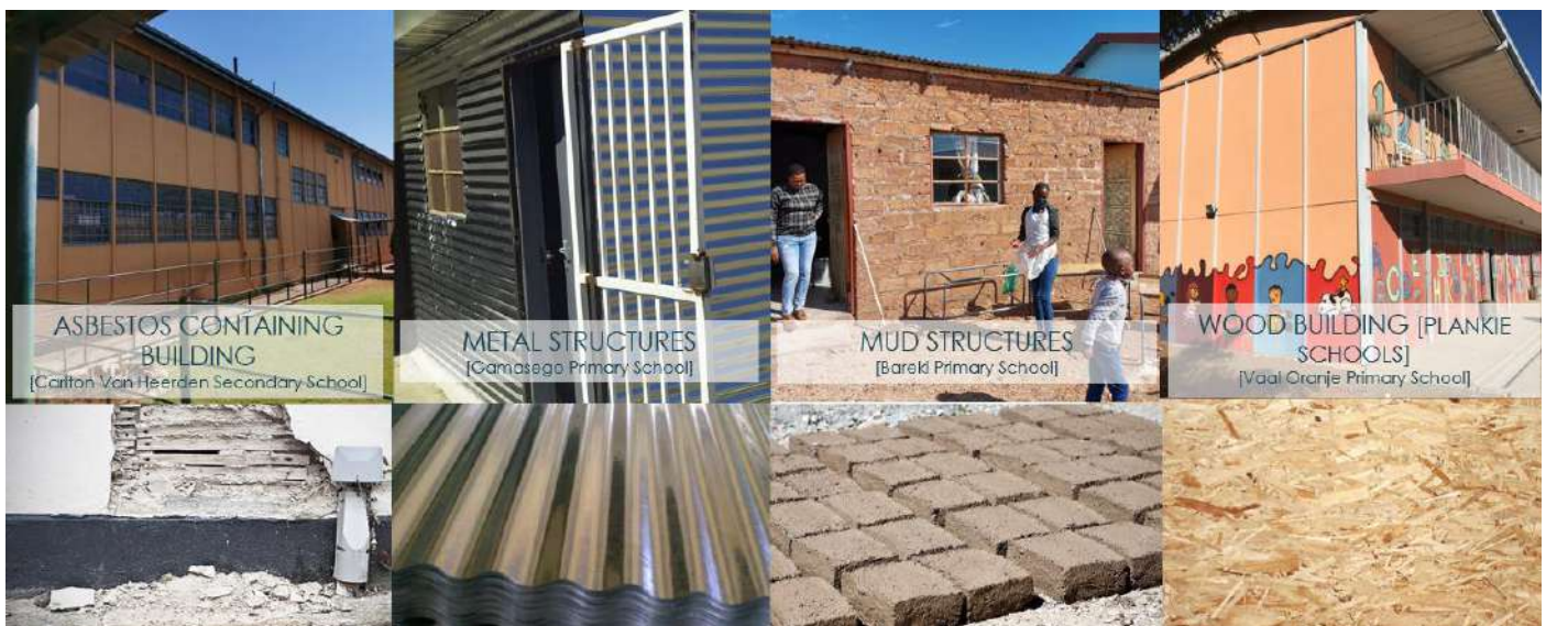
Figure 2: Inappropriate Structure Examples
